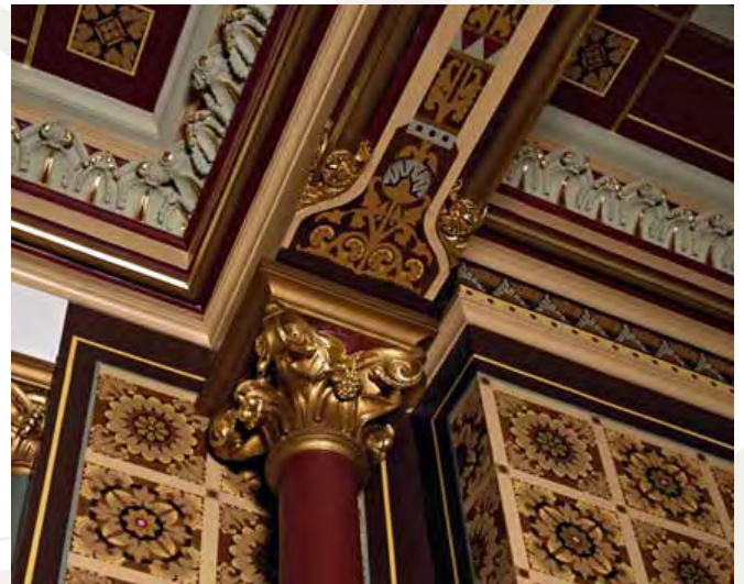
Connecticut Capitol. Photo courtesy of John Canning & Co., Decorative Painting and Restoration Contractor Photo Credit: © Robert Benson Photography
